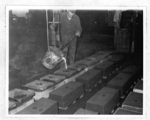
Figure 6. Pouring Ductile Iron Castings.
