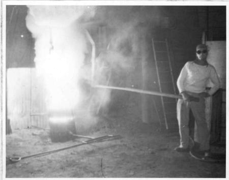
Figure 2. Two Views of Magnesium Addition to Ductile Iron.
