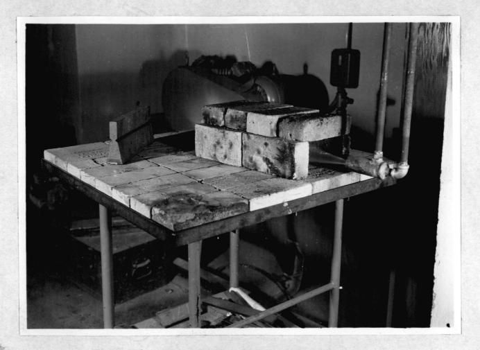
Figure 26. Table and Burner for Preheating Castings.
