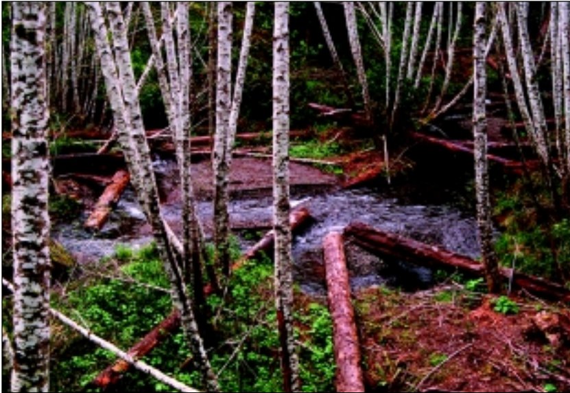
Figure 18.—Large wood being placed in the stream channel and floodplain of Beaver Creek in Curry County, OR. (Photo: Derek Godwin)
