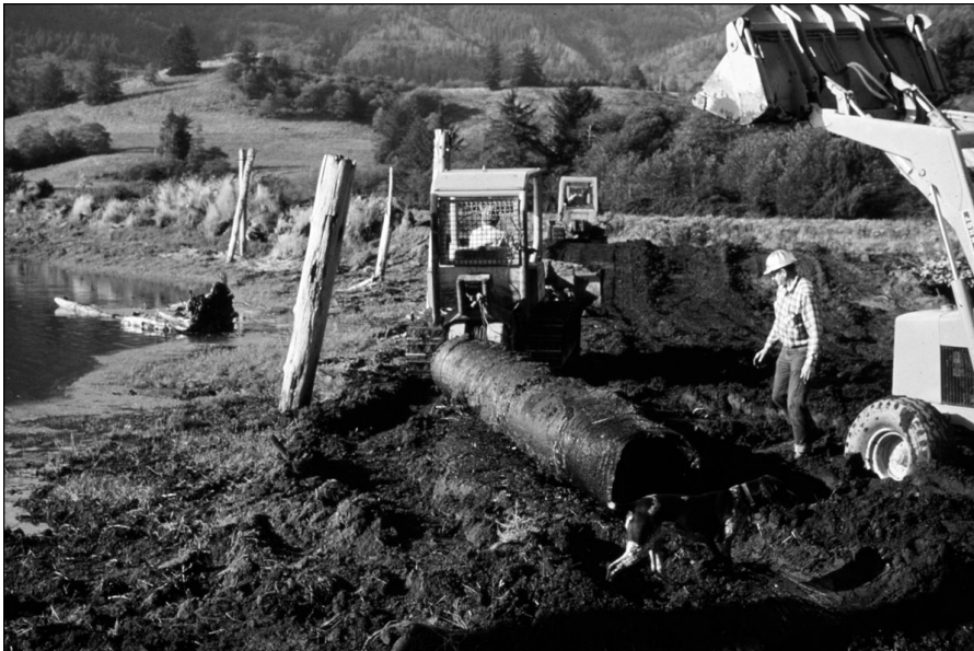
Figure 5.—Dike and tide gate removal in a 1978 Salmon River estuary restoration project opens up tidal channels that provide important rearing habitat. (Photo: Diane Mitchell)
