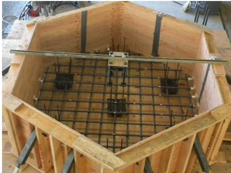
Figure 3.1.5b: Reinforcement placement and formwork for Pile Cap #7
