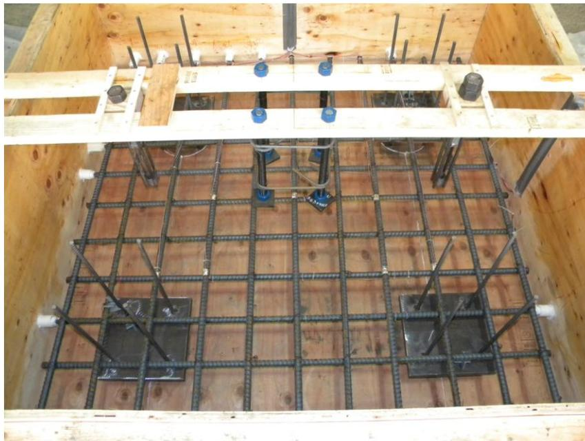
Figure 3.1.3b: Reinforcement placement and formwork for Pile Cap #4
