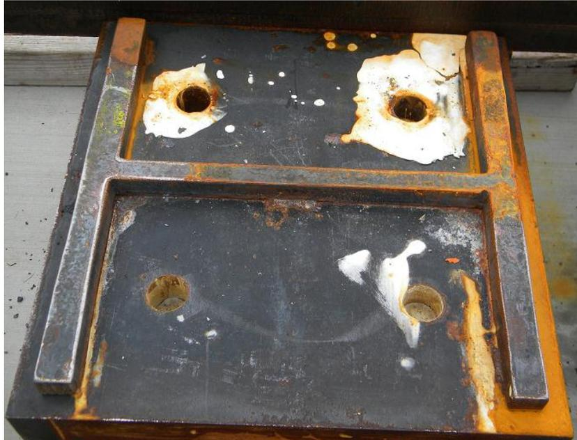
Figure 3.3.3: W14x99 profile attached to 3 in. bearing plate (note: white material is hydrostone used to grout baseplate)
