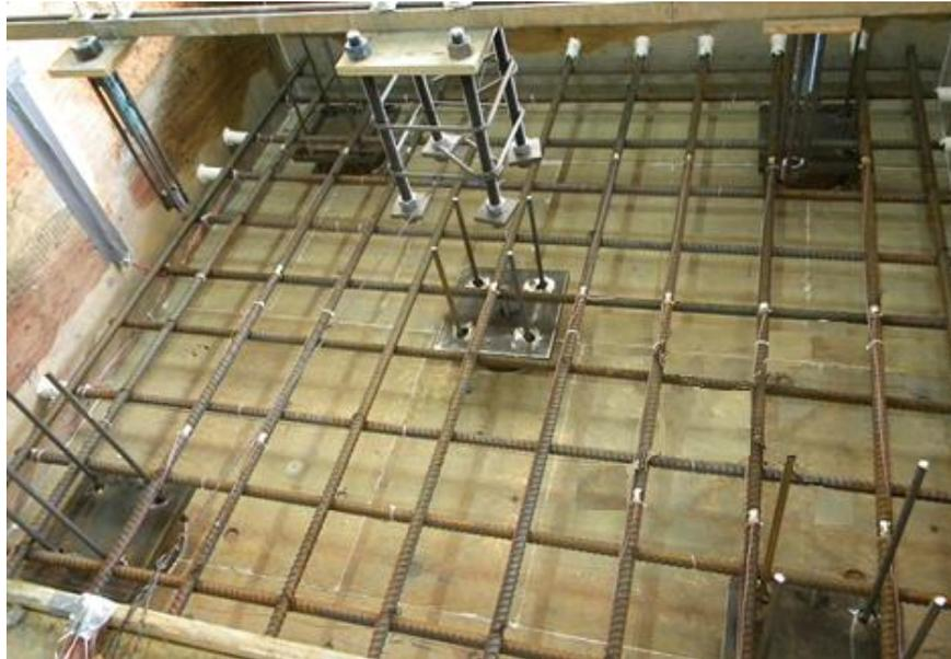
Figure 3.1.4b: Reinforcement placement and formwork for Pile Cap #5
