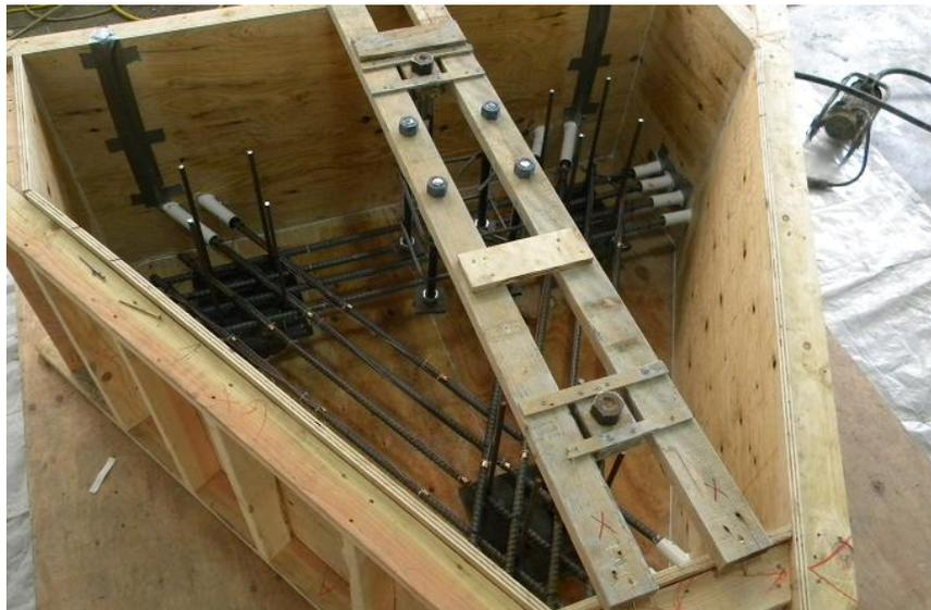
Figure 3.1.2b: Reinforcement placement and formwork for Pile Cap #3
