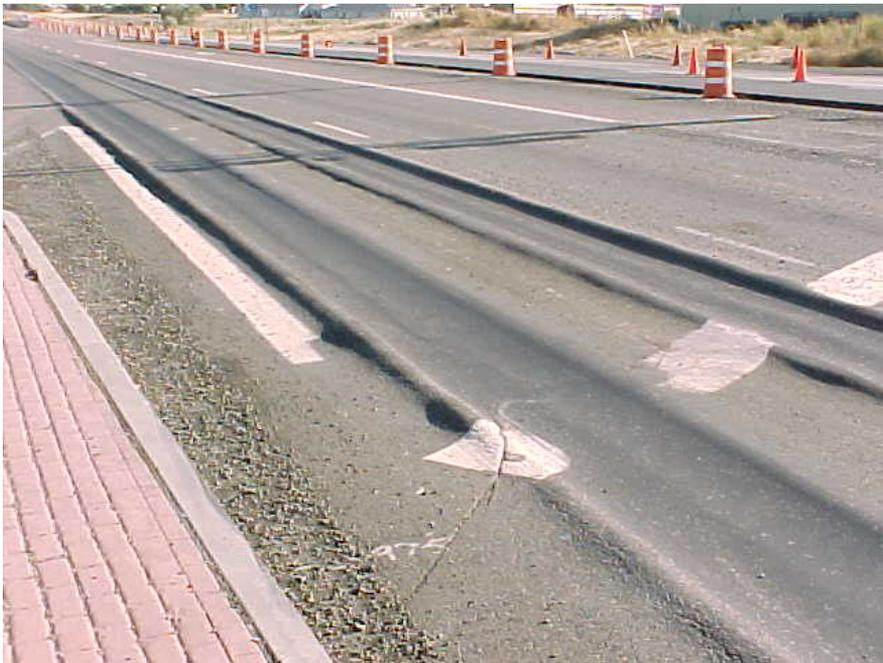
Figure 1.1 Permanent deformation
