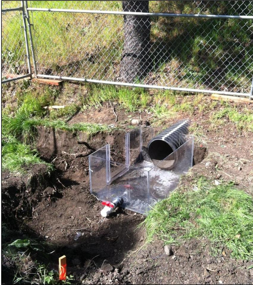
**Figure . Installed inlet structure**
