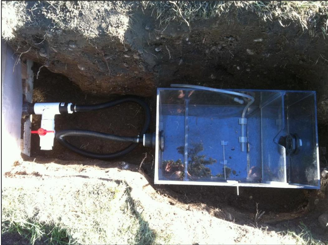
**Figure . Installed outlet structure**
