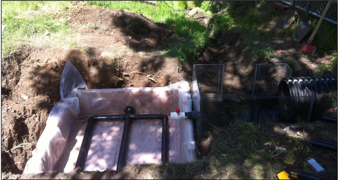
**Figure . Installed filter bed with polyethylene sheeting**
