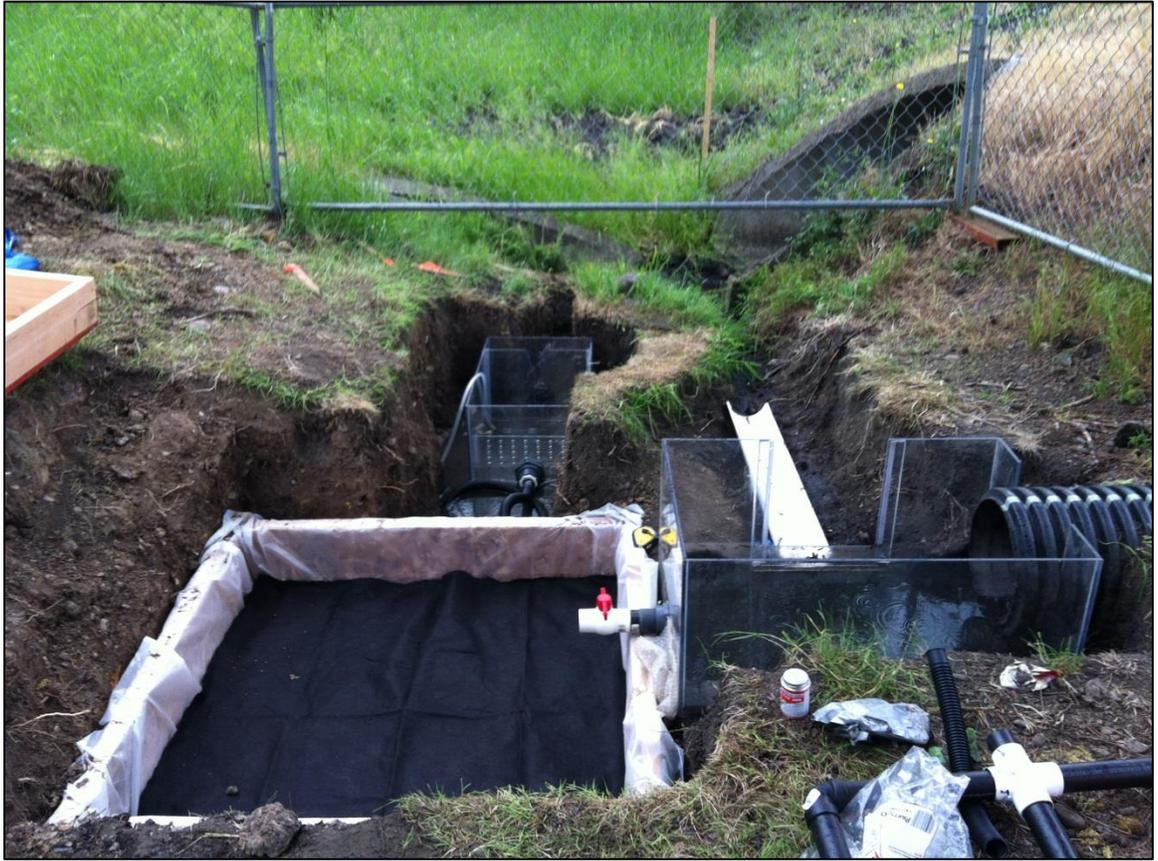
**Figure . Geotextile material installed between gravel and Apatite II™ layers**
