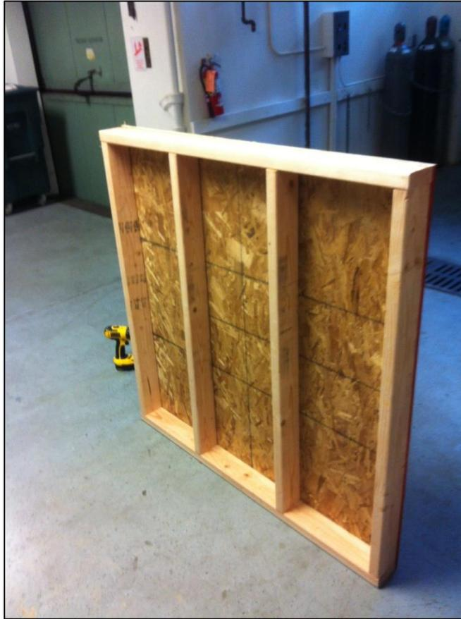
**Figure . Filter bed frame and floor**
