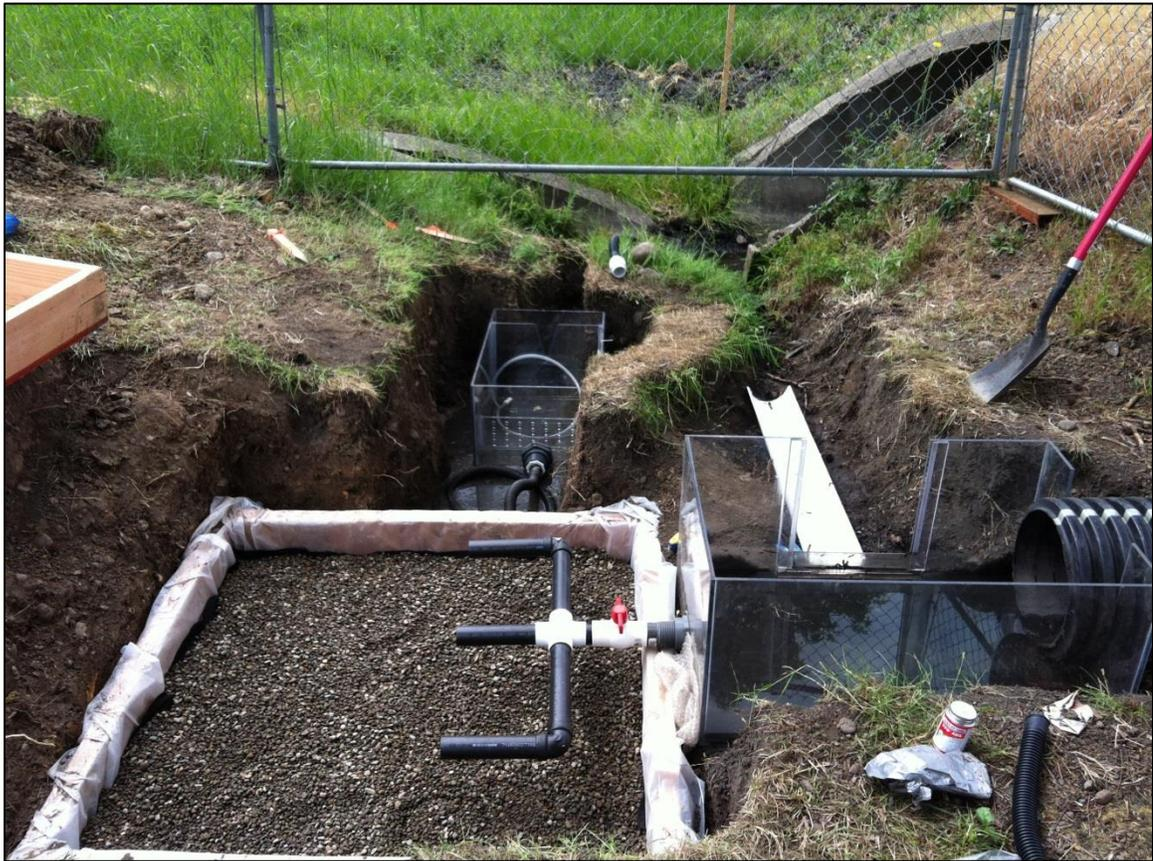
**Figure . Final gravel layer installed in filter bed**
