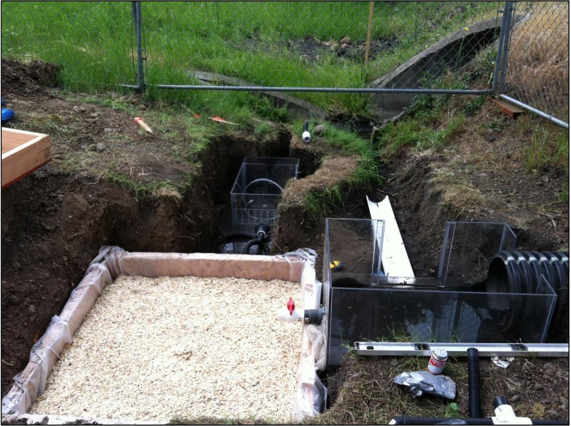
**Figure . Installed 4" layer of Apatite II™ media**
