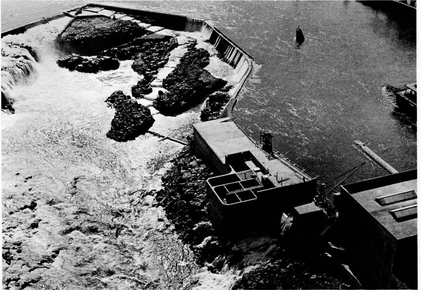
Cul-de-sac portion of the new Willamette Falls fishway (right-center) was completed during the biennium to replace the old inadequate ladder (upper-left) at Oregon City's historic barrier to migrating fish. A ladder constructed at the Falls in 1885 was the first such work ever undertaken in Oregon.
