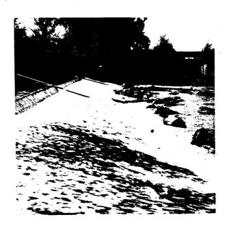
Figure 1. Inadequately laddered four-foot high dam on Coast Fork Willamette River, river mile 25.3.
