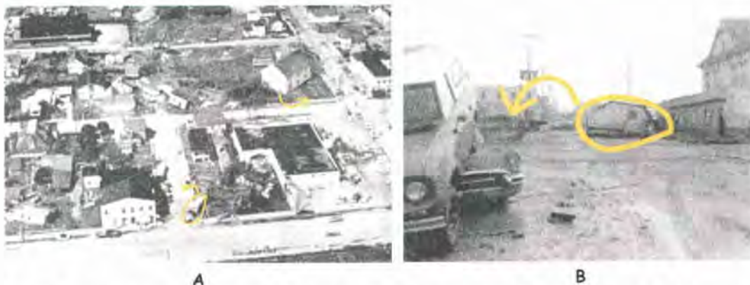
Figure 5-10: "Brass knuckles" of the ocean. The photograph of F and G Streets in downtown Crescent City (A) was taken two days after the 1964 tsunami surged onto the North Coast. Note the house in the upper left corner, shoved at an angle from its foundation. The semi-truck at the bottom center was shoved from the street onto the adjacent lawn. A close view of the streets of downtown Crescent City (B) also shows a car thrown onto another and a house ripped off its foundation (arrow). (Modified from Dengler and Moley, 1999)
