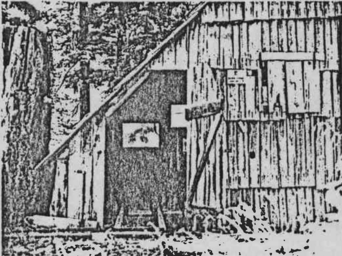
Building Made of Milled Lumber (photo courtesy Oregon State University)
