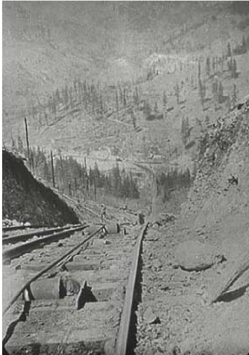
Figure 6.10: Looking down the Porter-Carstens incline in 1924 (Penn State University, group number MGN 103, box 32, folder 11).
