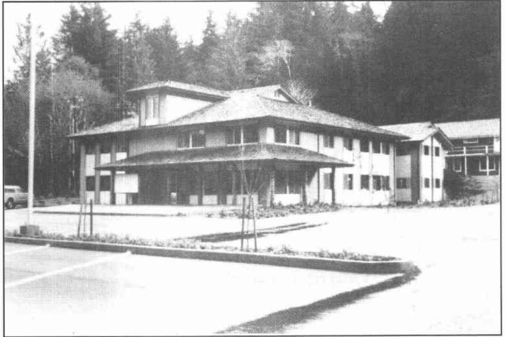
Figure 2-21. Quinault Ranger Station, Olympic National Forest, Region 6 (1974)
