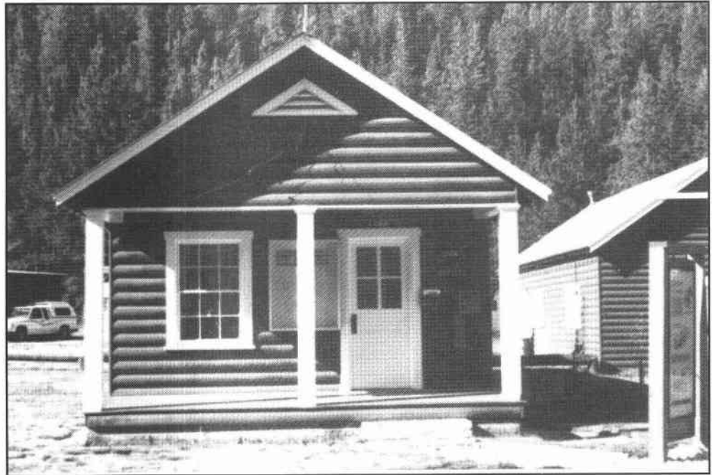
Figure 1-34. Warren Guard Station, Payette National Forest, Region 4 (1934)
