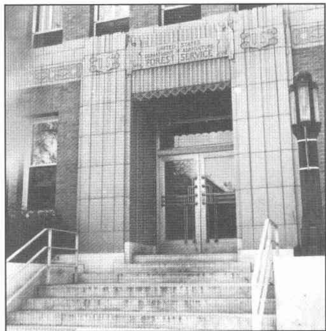
Figure 2-4. Entrance detail, Region 4 Office
