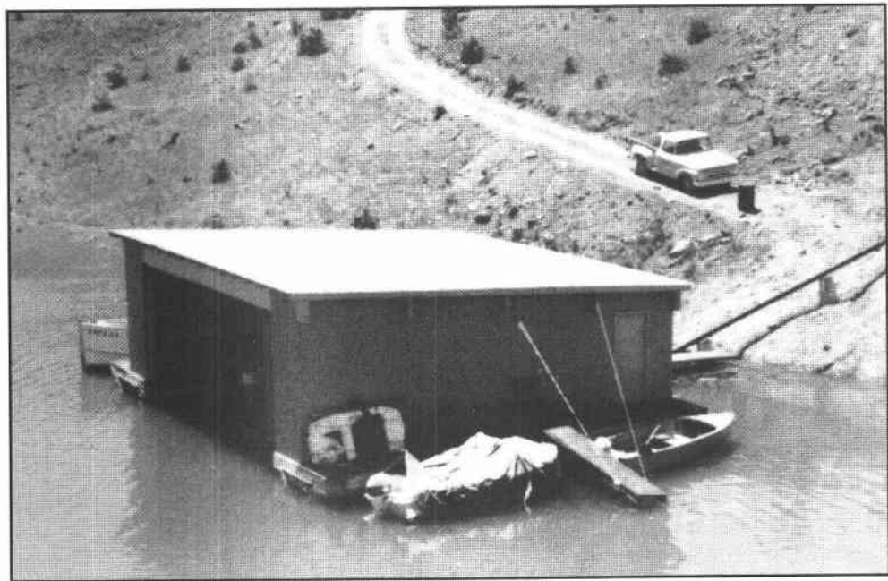
Figure 2-60. Mule Creek Boat Dock and Monorail, Shasta-Trinity National Forest, Region 5
