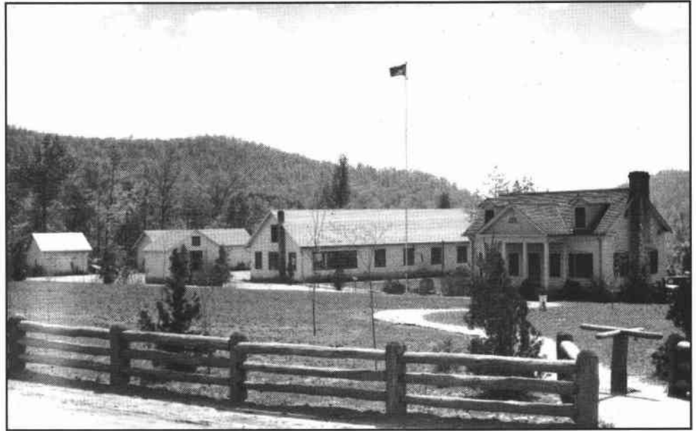
Figure 2-1. Blue Ridge Ranger Station Office and warehouse, Blairsville, Georgia
