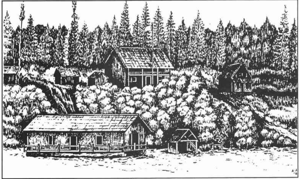
Figure 1-9. Boathouse, Priest Lake Ranger Station, Region 1 (1911)
