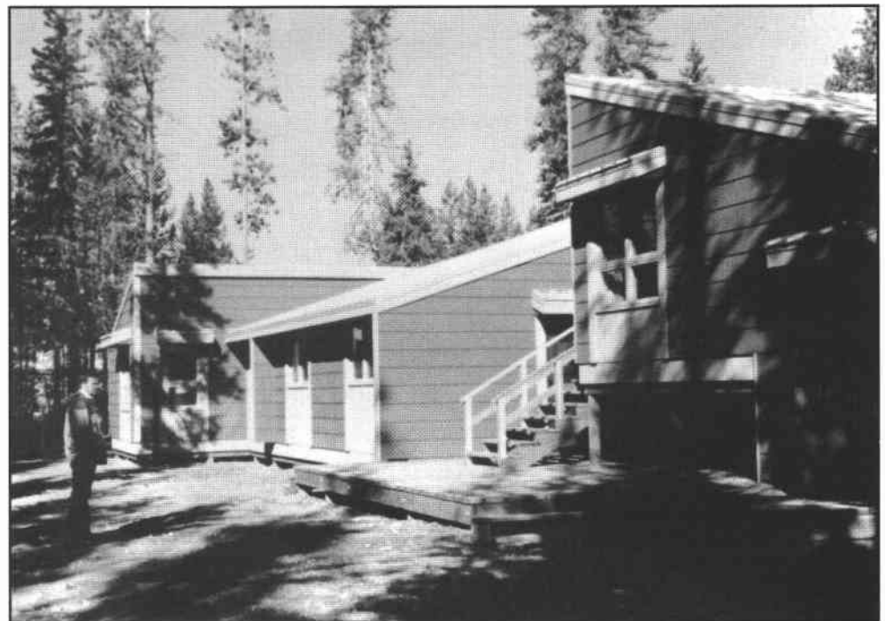
Figure 2-43. Ten-person barracks, Tyrrell Work Center, Bighorn National Forest, Region 2
