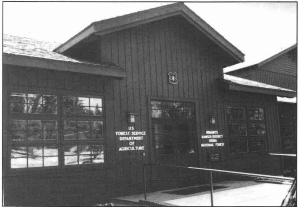
Figure 2-16. Minarets Ranger District Office, Sierra National Forest, California
