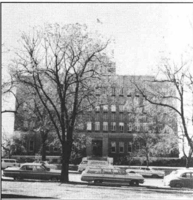
Figure 2-3. Region 4 Office, Ogden, Utah (1933)
