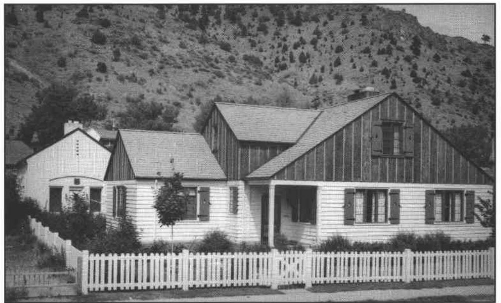
Figure 2-50. Supervisor's residence, Clear Creek Ranger Station, Arapaho National Forest, Region 2 (1939)
