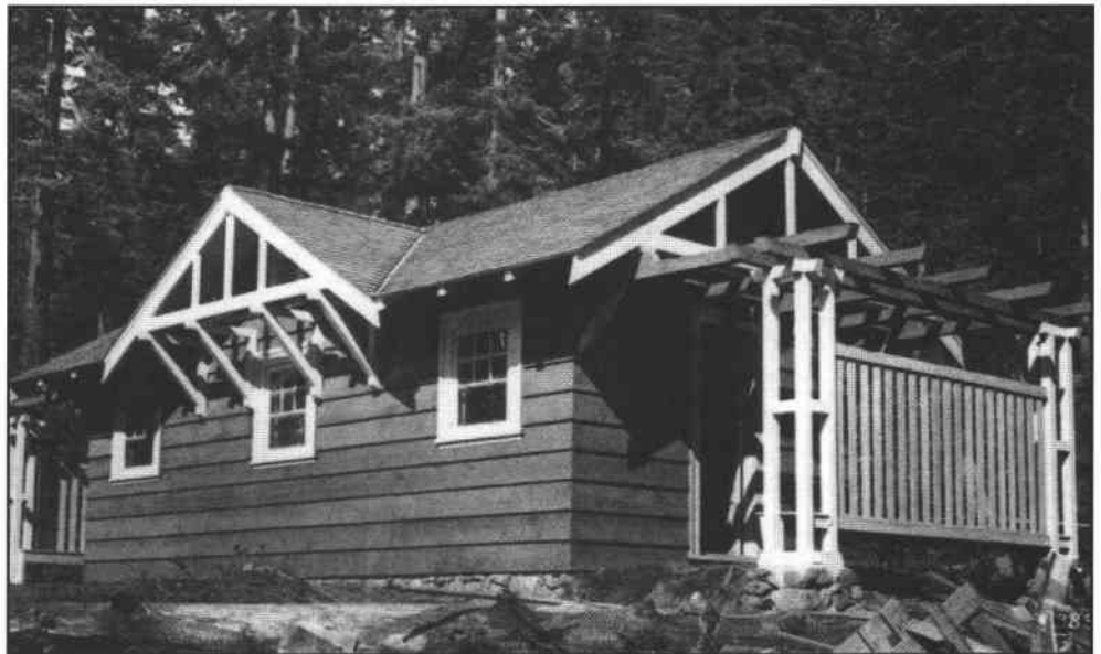
Figure 2-75. First substantial toilet building, Mt. Hood National Forest, Region 6 (1916)
