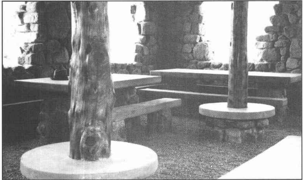
Figure 2-98. Interior detail of picnic shelter, Cibola National Forest, Region 3 (1936)
