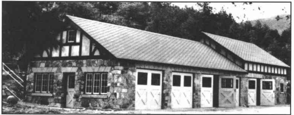
Figure 1-36. Crown King Ranger Station barn and shop, Prescott National Forest, Region 3 (1936)
