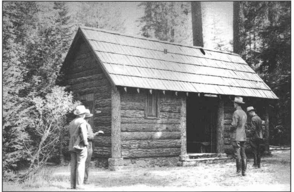
Figure 2-80. Combination toilet and registration building, Rogue River National Forest, Region 6 (1936)
