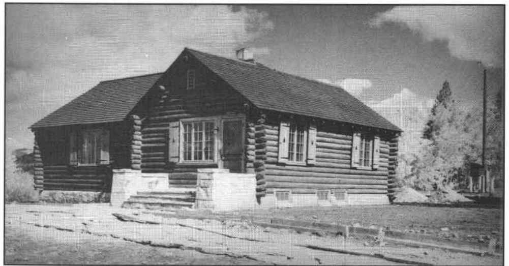
Figure 2-17. Brush Creek Office, Grand Mesa National Forest, Region 2 (1936)
