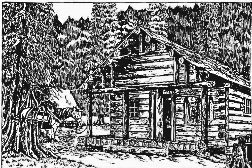
Figure 1-16. Twin Lakes Ranger Station, Region 1 (1924)
