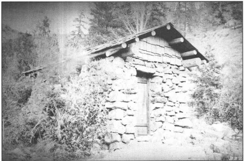
Figure 2-83. Toilet building, Chelan National Forest, Region 6 (1936)
