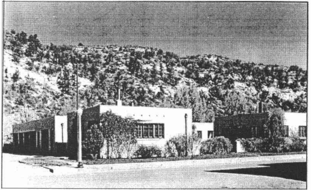
Figure 1-27. Delores Ranger Station, San Juan National Forest, Region 2 (1933-1938)
