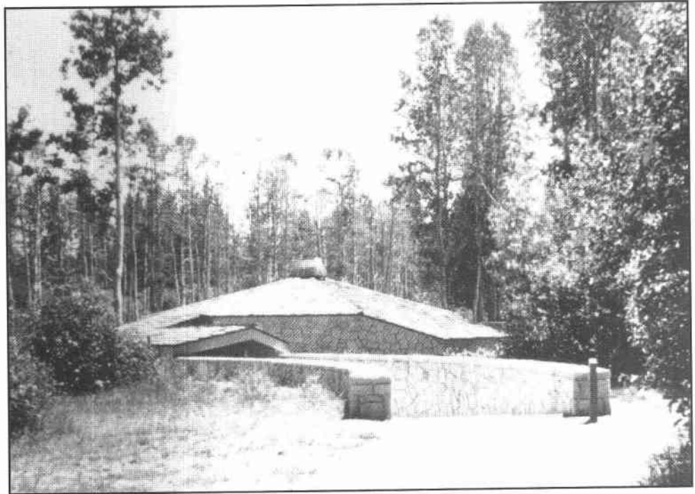
Figure 2-109. Stream Profile Chamber, South Lake Tahoe, California, Region 5
