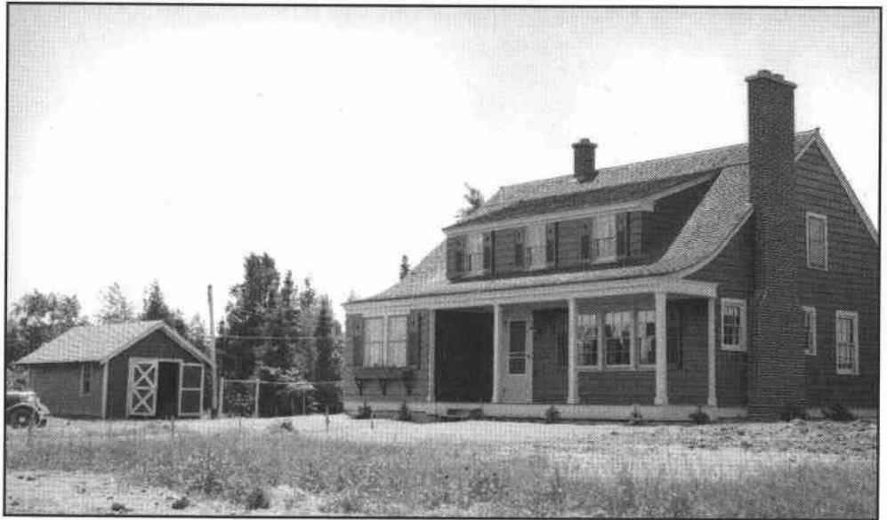
Figure 2-5. Ranger Residence, Pestigo Ranger Station, Nicolet National Forest, Region 9 (1936)
