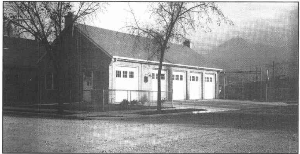
Figure 2-56. Cochetopa Warehouse, Salida Work Center, San Isabel National Forest, Region 2 (1938)
