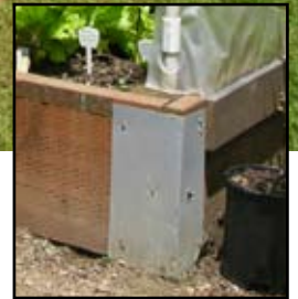
Figure 3 insert. Outside corner metal straps add stability to the raised-bed base.
