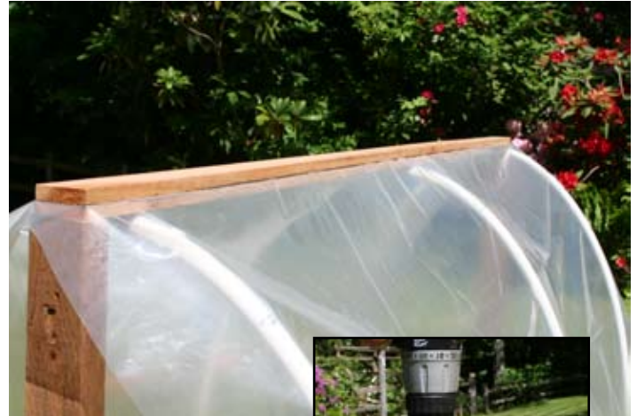
Figure 9. Sandwich and secure 10 x 10-foot plastic between the two D boards.
