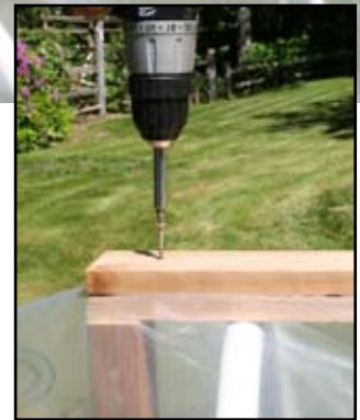
Figure 9 insert. Secure the plastic with 1.5-inch screws.
