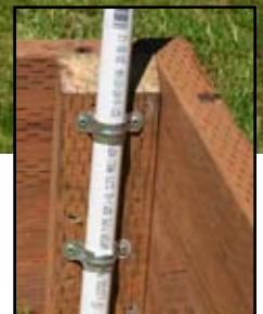
Figure 4 insert. Insert pipe straps.
