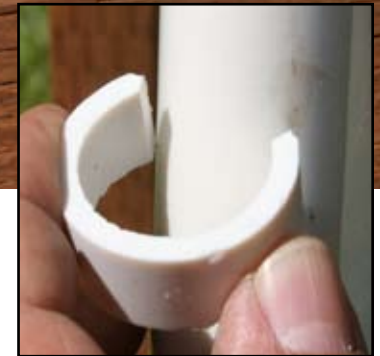
Figure 7 insert. Attach PVC clips to hoop.
