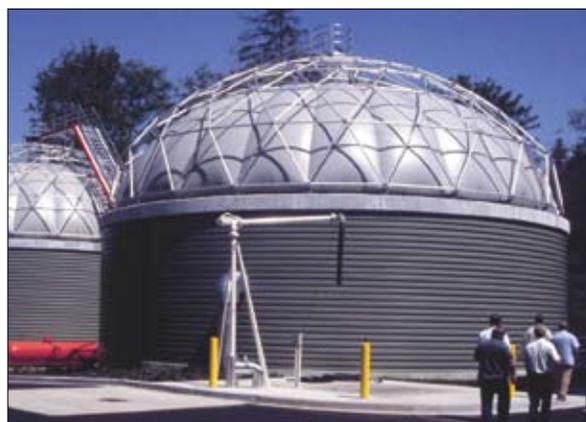
*At many treatment plants, anaerobic digestion in large vessels is used to process biosolids.*
