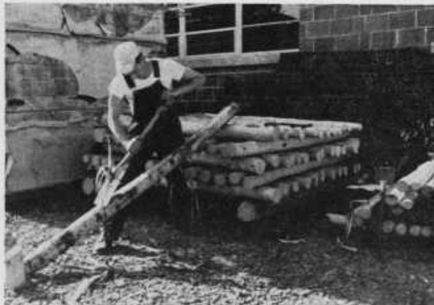
The bark must be completely removed from the post. Even small shreds of inner bark prevent absorption of the preserving solution. Plan your work so you can peel within a few days of cutting because drying causes the bark to tighten. A draw-knife is needed for a clean job when the bark is tight. During the easy-peeling season a straight spade or straightened goose-neck hoe makes a good hand peeling tool.
