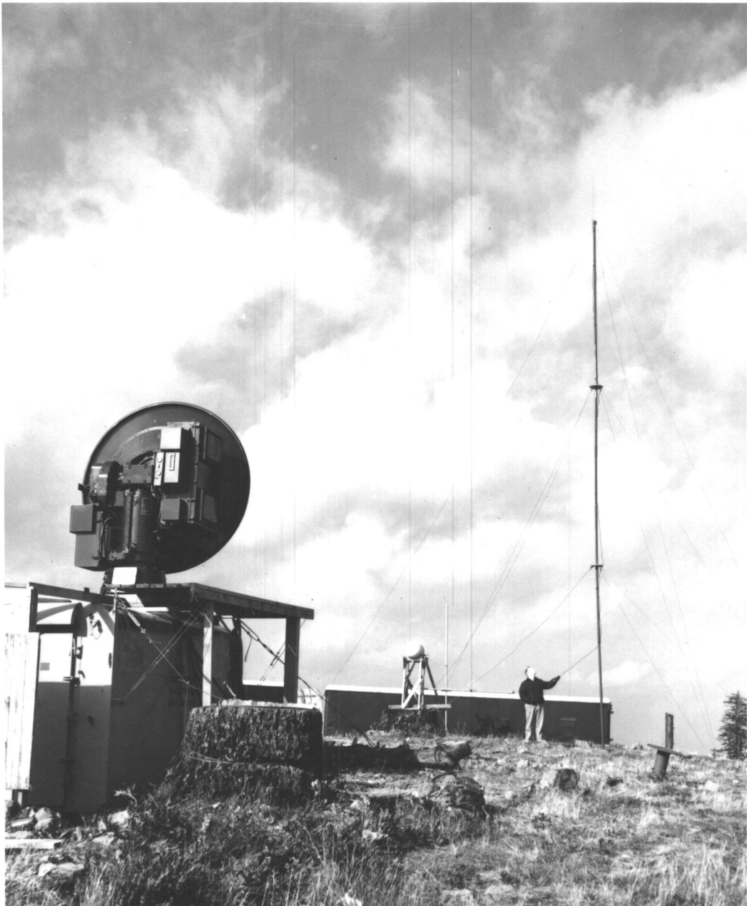
Fig. 7 RADAR ANTENNA AND POINT DISCHARGE ANTENNA ATOP McCULLOCH PEAK
