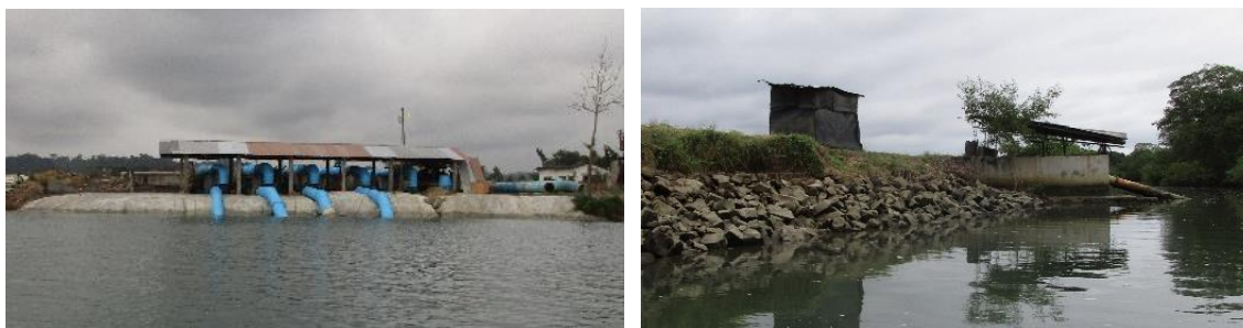
Figure 23: Water pumps connect shrimp ponds to waterways on the other side of a pond's wall.
