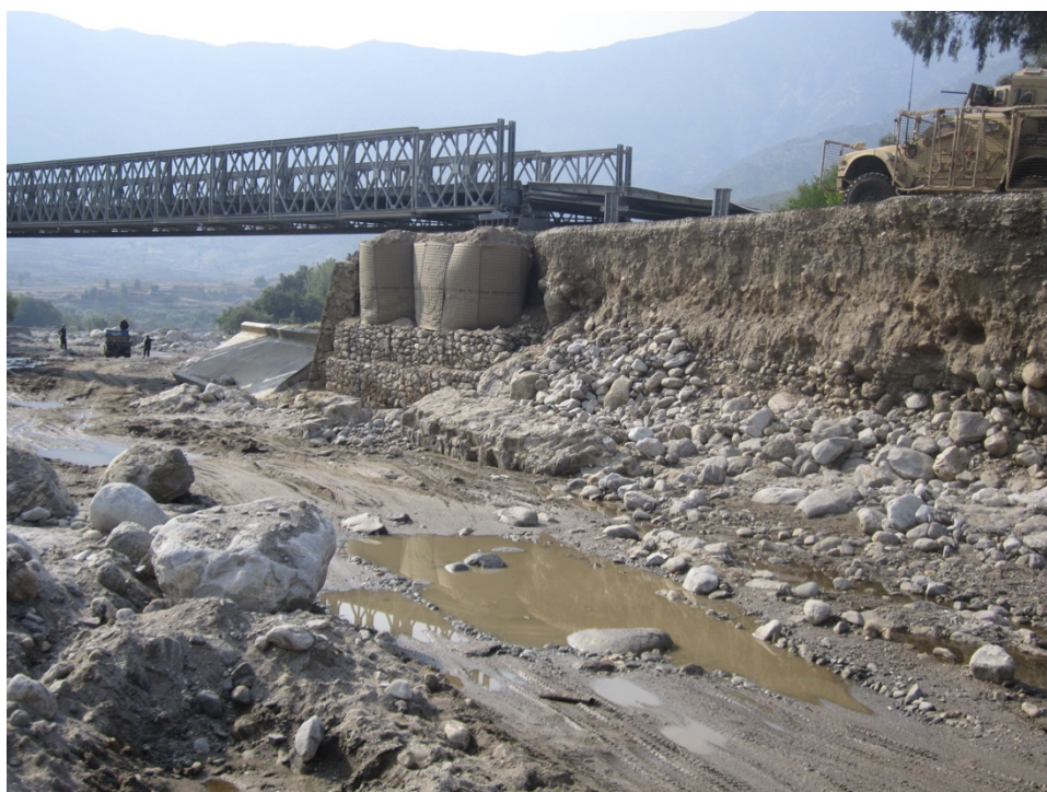
Figure 3.1. Photo of bridge emplaced over the Watapur River. Old concrete bridge is visible lying on the riverbed under the new bridge. Photo by author.
