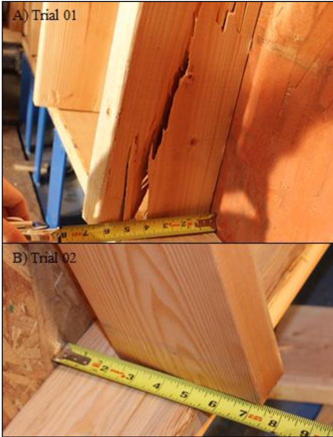
Fig. 15: FAIL1 failures: A) Trial 01 stud splitting, B) Trial 02 stud to bottom plate connection failure
