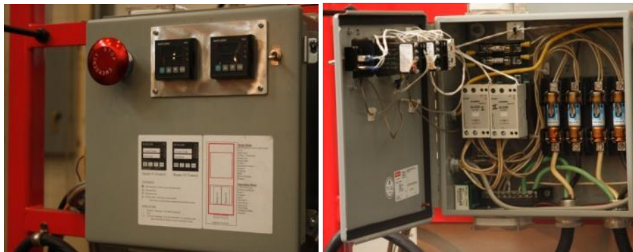
Figure 3.4-4: Picture of the heater control box. Left- exterior, Right- interior.
