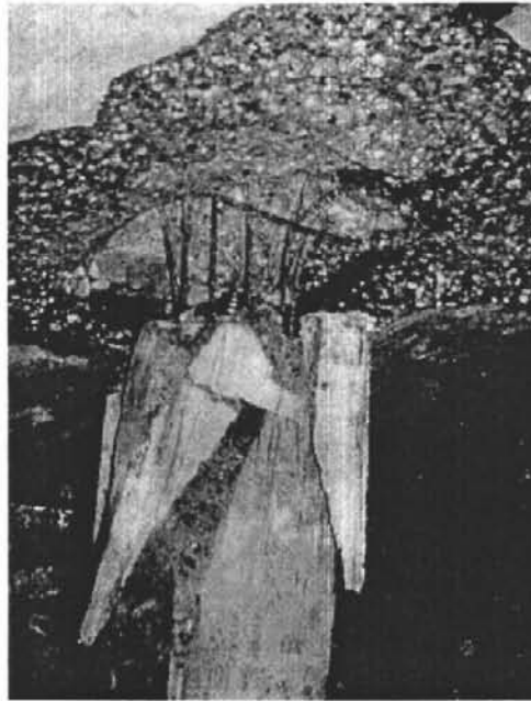
Figure 1-3: Batter pile/wharf deck connection damage, Port of Oakland, 1989 Loma Prieta Earthquake (Werner, 1998)
