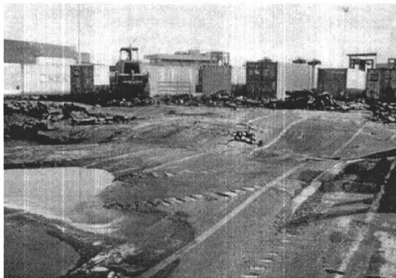
Figure 1-4: Post-liquefaction settlements at Matson Terminal, Port of Oakland, 1989 Loma Prieta Earthquake (Werner 1998)
