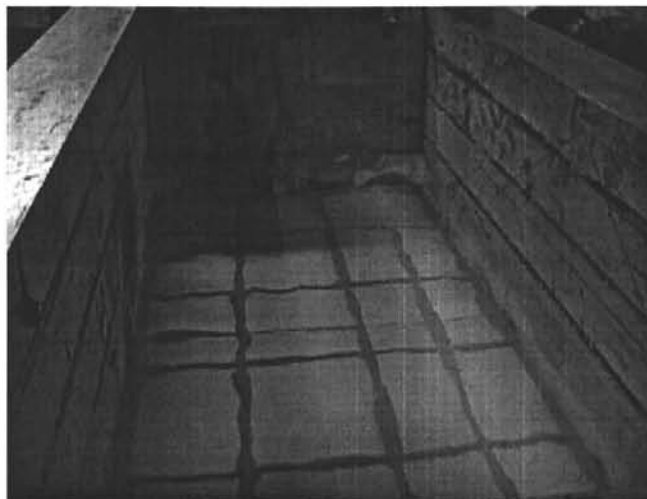
Figure 5-5: Drainage layer between clay sub-layers
