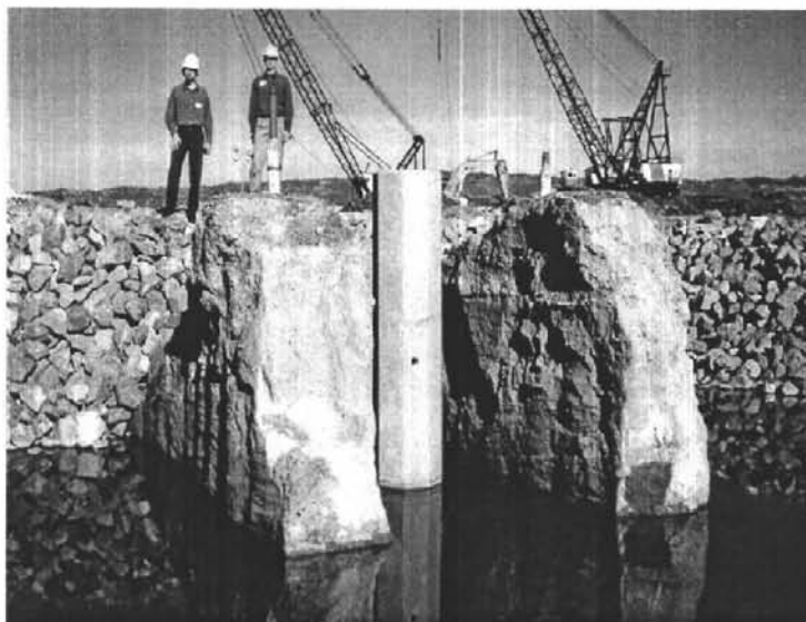
Figure 3-10: Test pile at Port of Oakland surrounded by CDSM material
