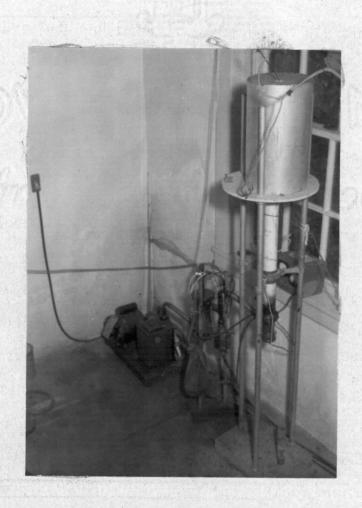
Figure 6. Electric Vacuum Furnace used for Alloying Magnesium with Zirconium.
