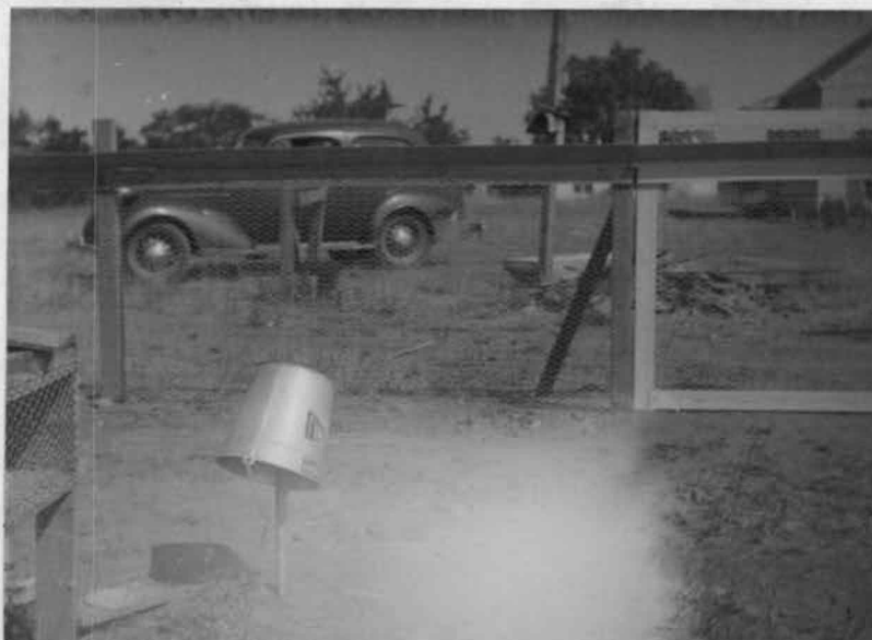
Fig.3 - This picture illustrates the use of a wire guard fence with a tin overhang.
