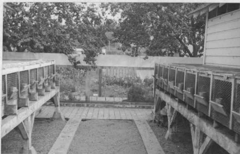
Fig.5 - The guard fence is 4 ft. high and of 16 gauge 1 in. mesh wire with a 12 in. piece of galvanized tin on top. The house and runs are all built on the same joists. The stringers can be seen at the end of the runs.
