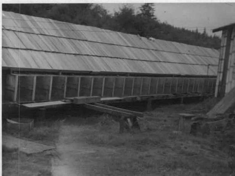
Fig.4 - This is an example of a modified type of Alaskan breeder house. The mink are in runs on wire floors. They are fed and watered inside. The small portion of the pen extending outside allows the mink to sun itself.
