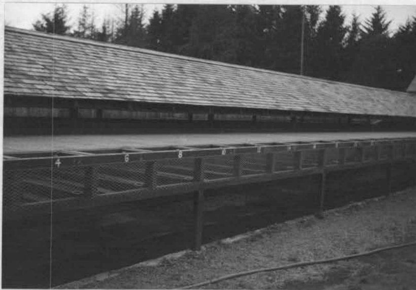
Fig.10 - This breeder house is neatly built with a concrete floor under the runs to facilitate cleaning. Water cans can be seen in front. A piece of plate glass in the run serves as a feed board.
