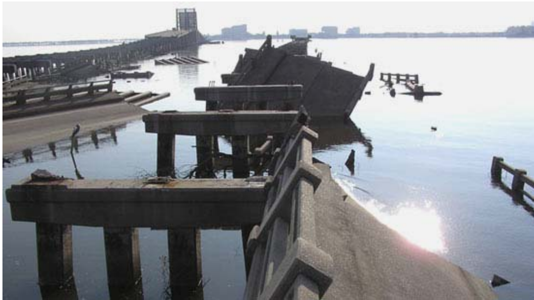
Figure 1-2. Damage to the U.S. 90 Biloxi Bay Bridge caused by Hurricane Katrina (courtesy of Solomon Yim, Oregon State University).
