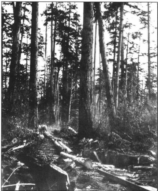
Gravity chute bringing logs down to a landing, ca. 1880s.
