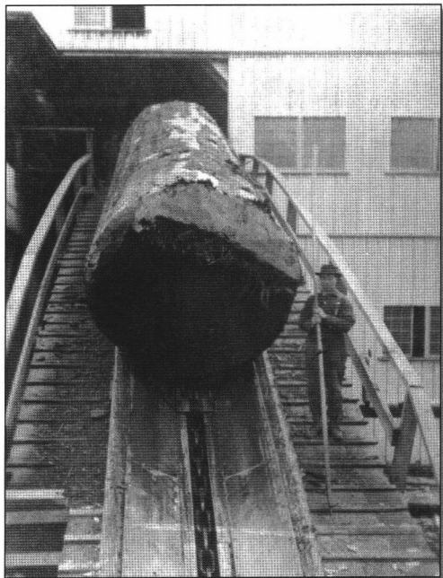
Log on bull chain, C.A. Smith mill, Coos Bay. C.P. Cronk photo, 1910-1911.
