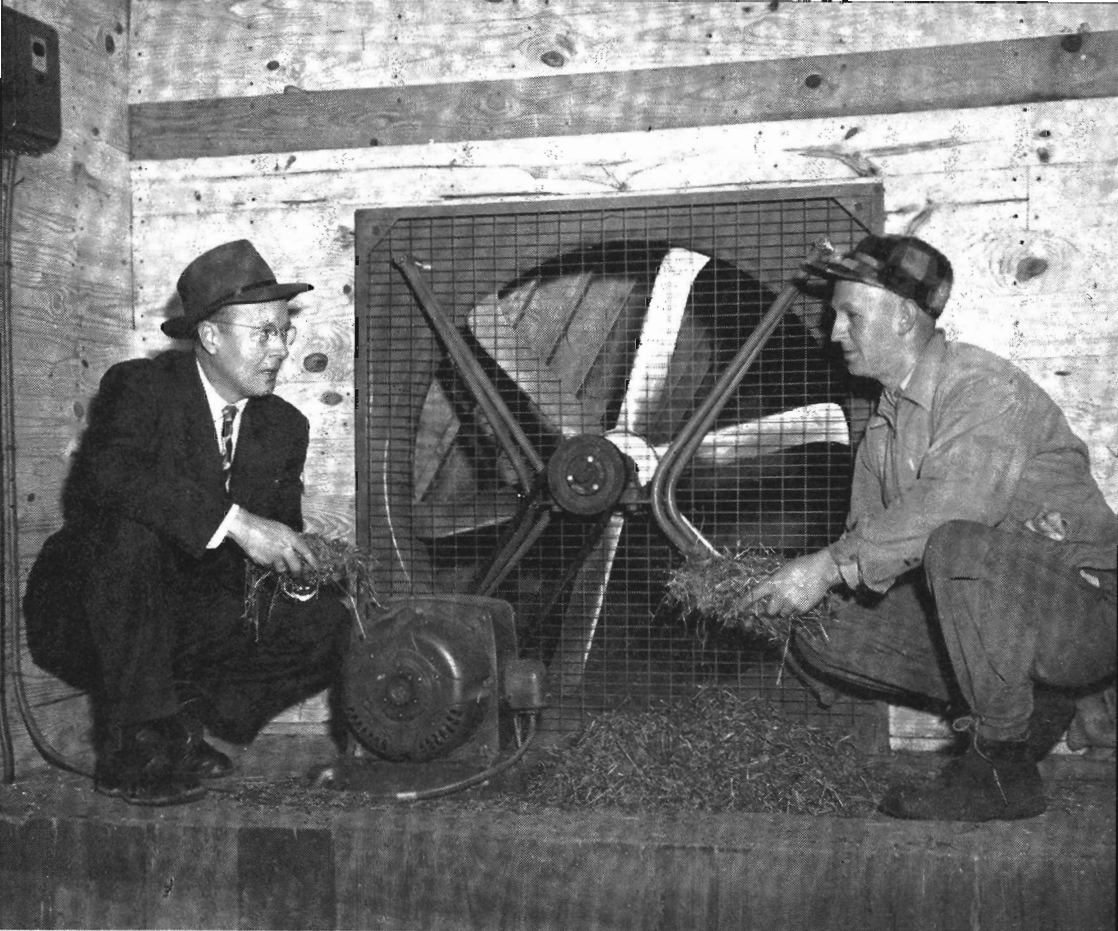
Figure 36. Six-blade, 36" propeller-type fan properly installed in an A-frame duct. Note the safety screen for the protection of personnel and the fan itself.
