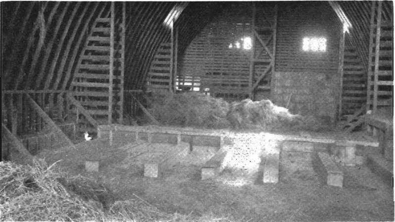
Figure 7. Lateral-duct system with center main servicing one end of a large mow. Top , the drier with a load of hay in place. Bottom , the duct system after the hay has been removed.
