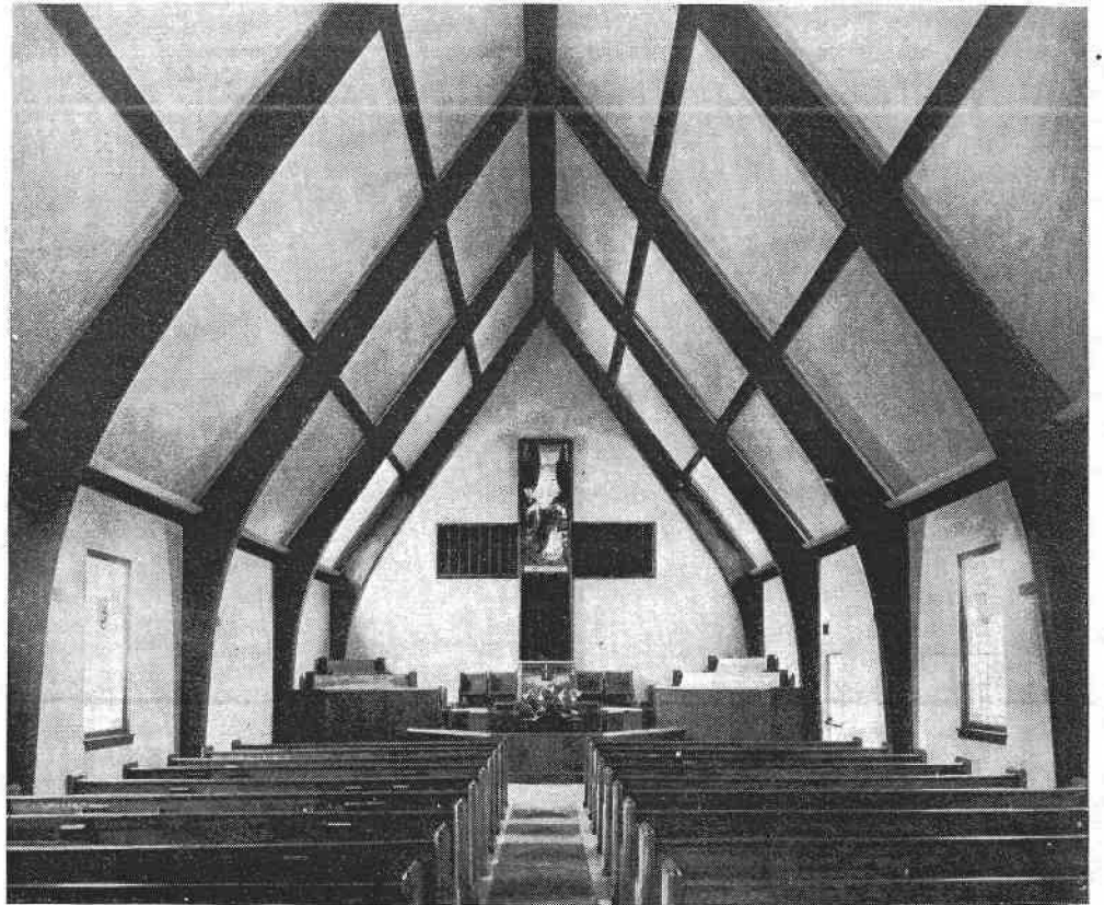
FIGURE 9.—United Brethren Church at Seattle, Wash. Width, 32½ feet; height of glued laminated arches, 36¾ feet.
