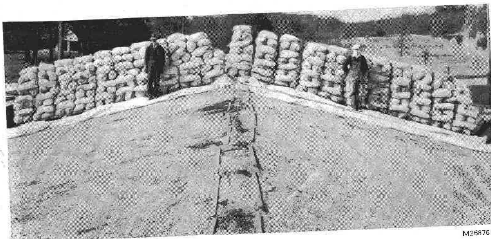
FIGURE 42.—Sandbags on central arch span of Forest Products Laboratory service building.
