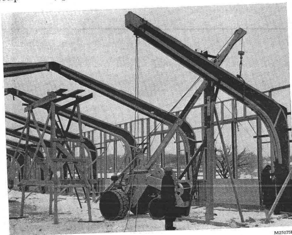
FIGURE 41.—Erection of arches in Forest Products Laboratory service building.
