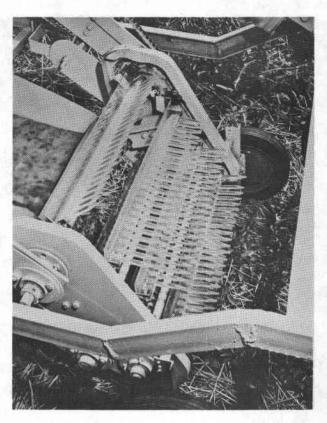
Figure 5. The stripping mechanism of the University of Illinois harvester originally had plastic fingers. [Photograph courtesy of Dean L. Hoag (23)].
