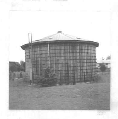
Figure 1. Redwood water storage reservoir; 50,000 gal capacity (189,400 1).
