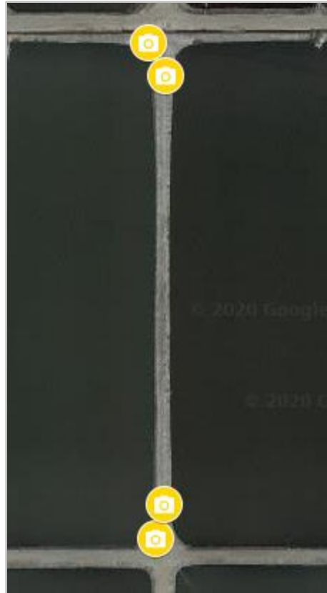
Figure 7: Locations of perimeter cameras at American Electric Power – South Dike. Each camera icon represents one camera.
