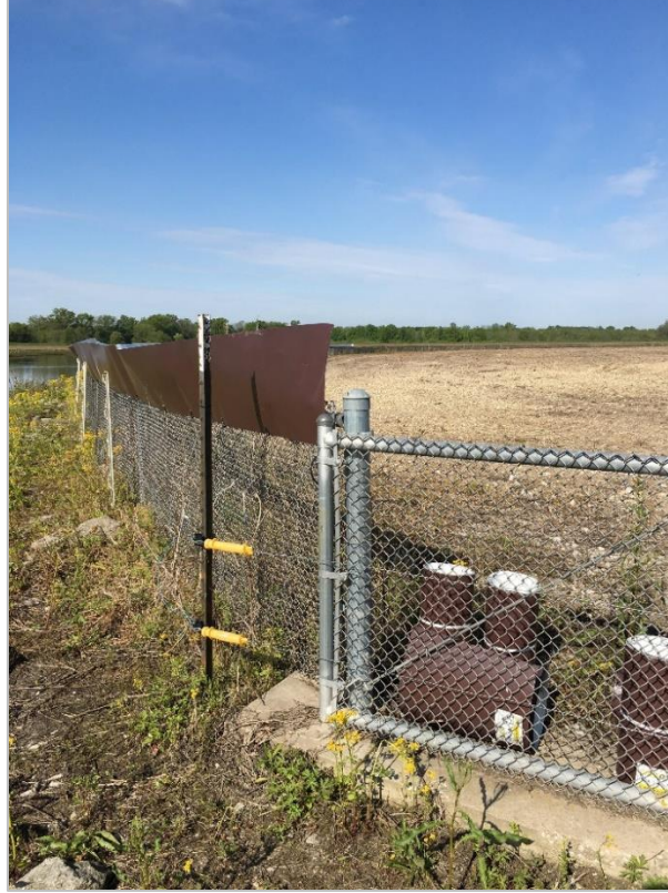
Figure 4: Exclosure with aluminum flashing on top of chain link fence at Goose Pond Tern Island, southern Indiana. Exclosure at Cane Ridge is the same but without the aluminum flashing.
