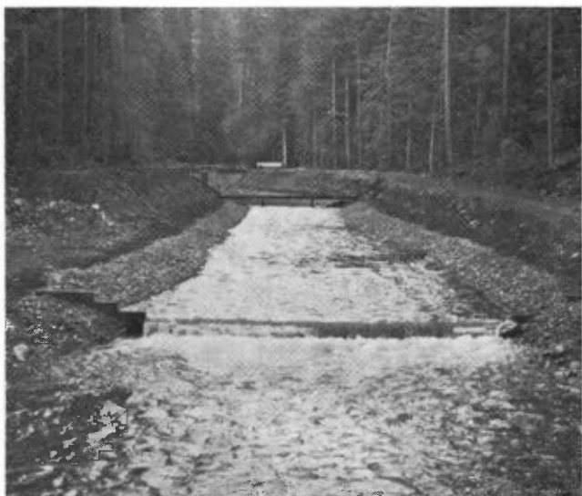
Artificial spawning channel at the Eugene Water and Electric Board's Carmen-Smith hydroelectric project on the upper McKenzie River. This 100-yard long channel is capable of accomodating about 200 spawning spring chinook salmon.
