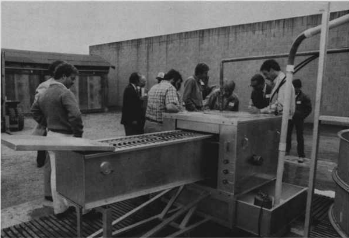
The automated squid cleaning machine developed by the Squid Machine Corp., Santa Cruz, California. Photo by Ken Hilderbrand.
