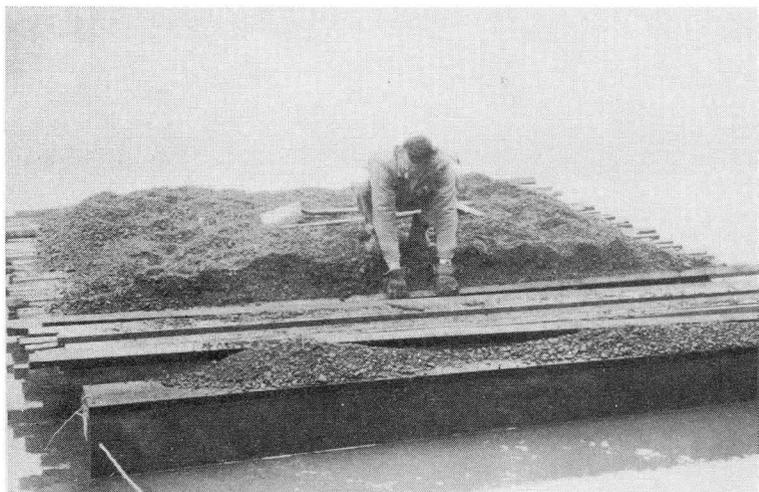
Fig. 10 Gravel being unloaded from barge by tipping
