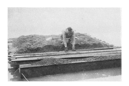
Fig. 10 Gravel being unloaded from barge by tipping 2 x 4  $^{\circ}$ s.
