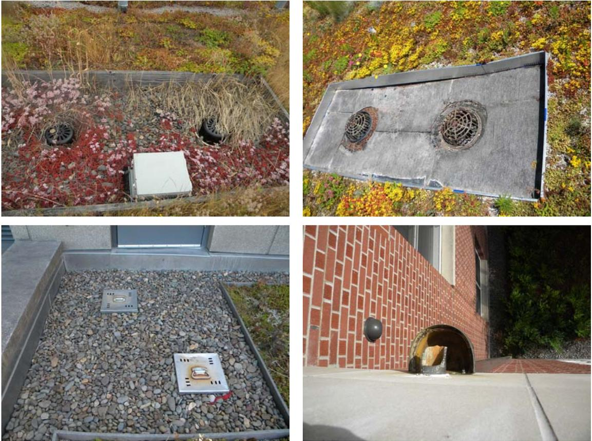
**Figure 1.3: Various encountered interior and exterior ecoroof drains.**
