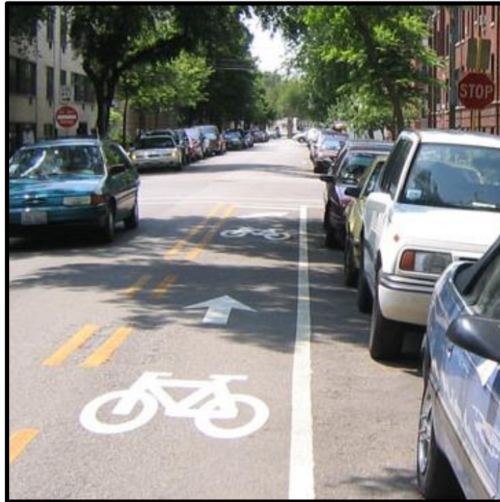
Figure 5.2: Example of a Contra-Flow Bicycle Lane in Chicago, IL (NACTO, 2011)
