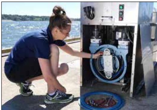
In a training video for maintenance staff, Jenny East demonstrates how to winterize the pump in a facility where boaters pump out their onboard sewage. (Photo by Vanessa Cholewczynski)
