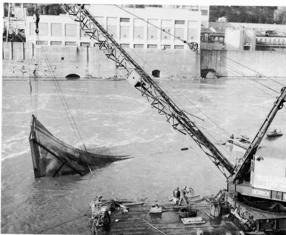
A giant net is lowered into place below the outlet of a turbine to catch downstream migrant steelhead and salmon. This operation was part of a study carried out by Game Commission biologists to determine mortality on these young fish.
