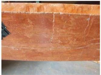
Figure 2: Damage to the right of taped area also caused by police boat accident
