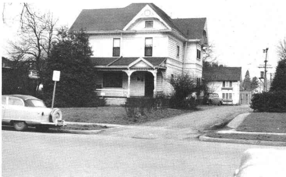
The Midgley-Hollenbeck-Grimes pioneer house, 245 E. 8th Ave. of particular interest at present—to be razed (or moved?) soon to make way for Eugene's new city hall. Built by George Midgley, (1881—founder) of Midgley Planing Mill. (#120-H) See also picture of double wedding held in this home, opposite page.
