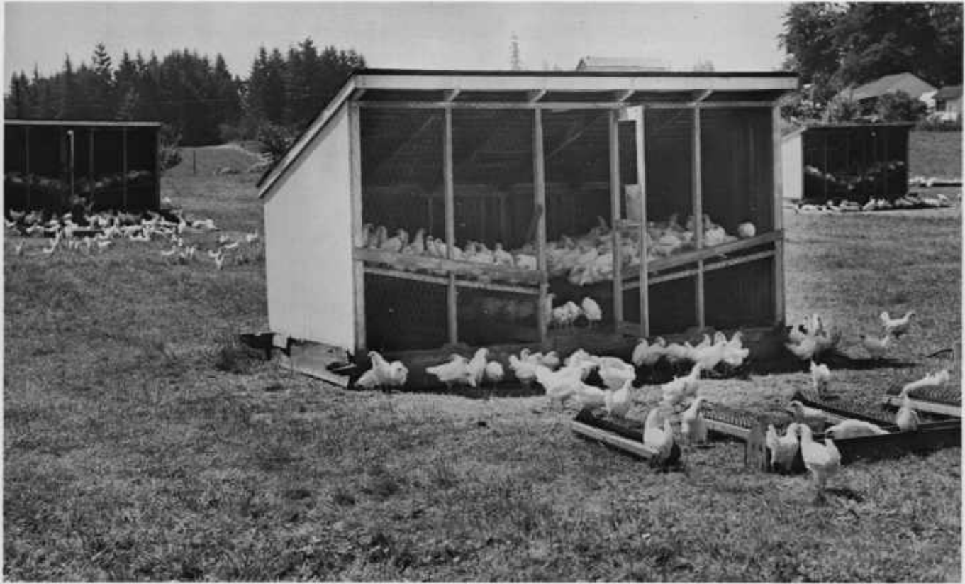
Figure 5.— Portable range shelters are built on skids so they can be moved frequently to new locations, reducing contamination.
