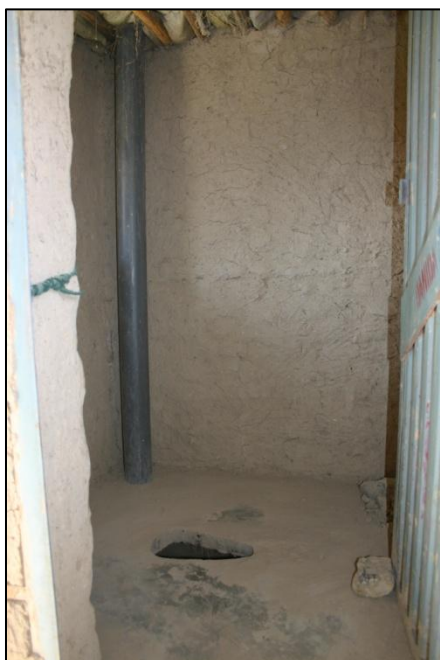
Figure 3.4: The inside of a ventilated pit latrine.
