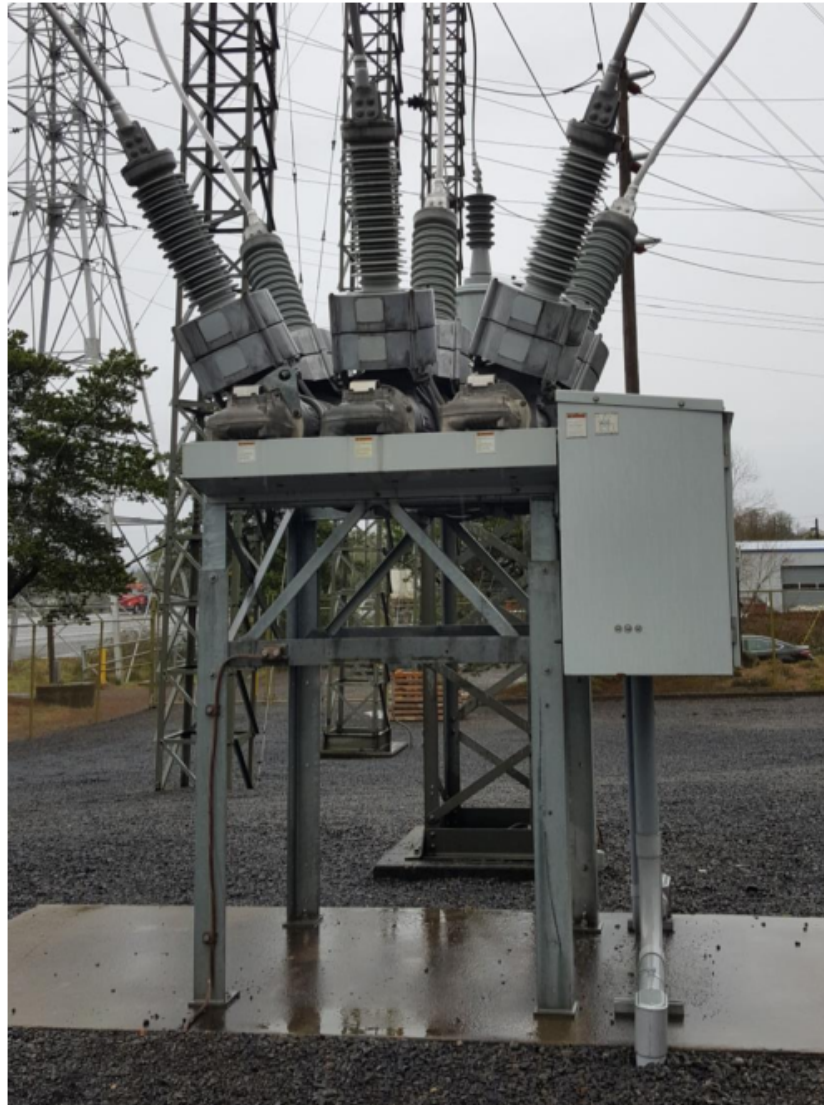
Figure 1.4: Circuit Breaker, Gas, 57 kV[2]
