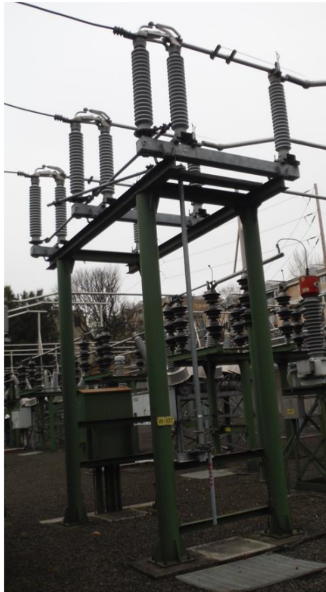
Figure 1.3: Disconnect Switch, 115 kV[2]
