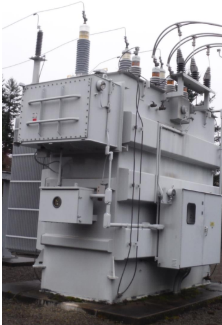
Figure 1.5: Transformer, 57 kV[2]
