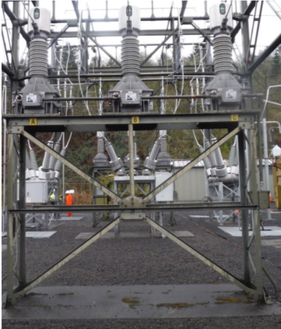
Figure 1.6: Current Transformer, 57 kV[2]
