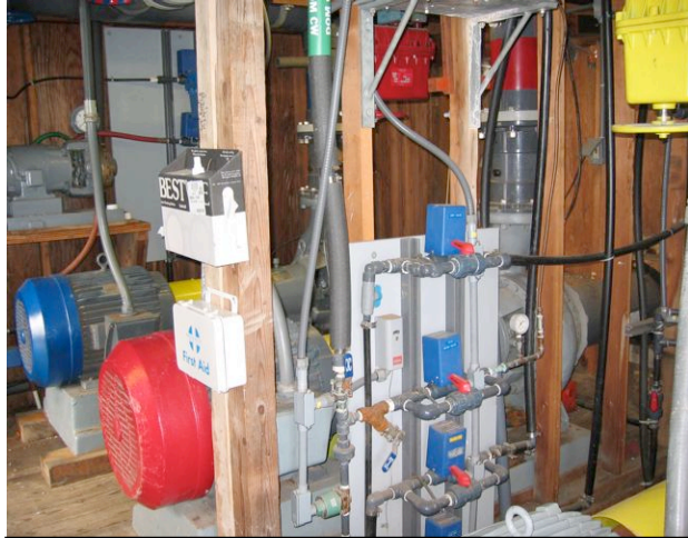
Figure 2: Inside the pumphouse showing two of the four seawater pumps.
