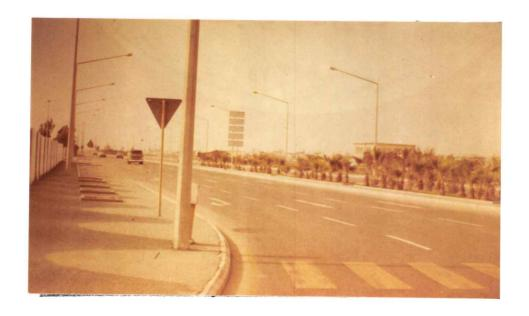
Figure 2.18. Green asphalt emulsion used for sidewalk and median treatment. "JEDDAH"
