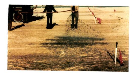
Figure 2.13. Emulsified asphalt spray mulch for seed protection. "JUBAIL"
