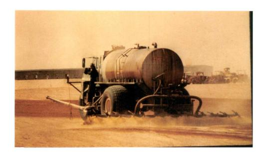
Figure 2.16. Asphalt emulsion (brown) spraying for sand stabilization. "JUBAIL"
