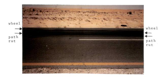
Figure 2.8. Pavement rutting due to high axle loads.
