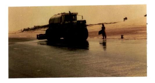
Figure 2.14. Fog sealing operation for surface protection. "JUBAIL"
