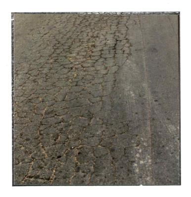
Figure 2.7. Subbase rutting, causing excessive surface failure.
