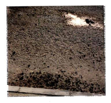
Figure 2.5. Aggregate disintegration.
