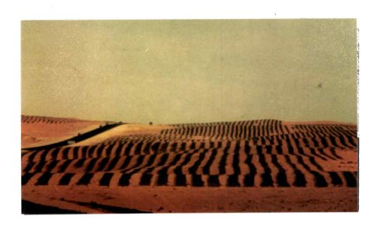
Figure 2.10. Sand dune stabilization to protect roads. "Al Majma'ah highway"
