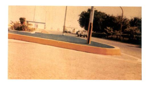
Figure 2.17. Dark blue asphalt emulsion used for median treatment. "JEDDAH"
