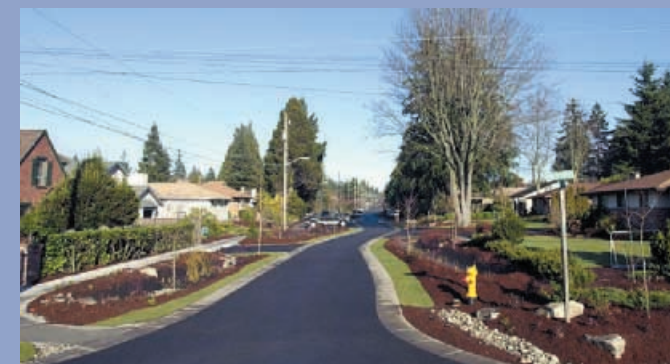
This residential street was redesigned by the City of Seattle under the Seattle's Street Edge Alternatives Program. Streets were narrowed and gutters removed so that runoff can be directed to swales and bioretention areas. (Photo courtesy of Seattle Public Utilities)
