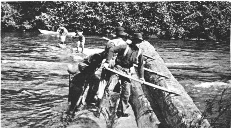
**“Driving” logs down the McKenzie River during pioneer days. Only trees near the rivers were felled and skidded to the banks by ox teams to be floated down to the sawmills during the spring freshets. Much hand labor was necessary to keep the logs moving — over the shallow gravel bars and when log “jams” would have to be dislodged.**
