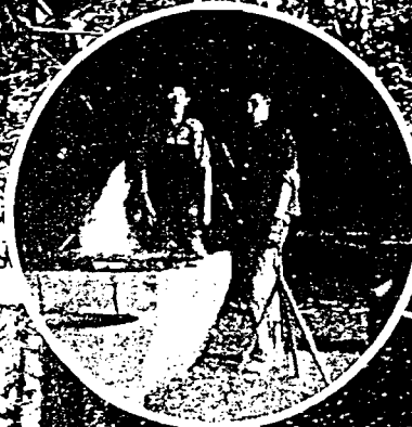
Making Culvert from Tree
