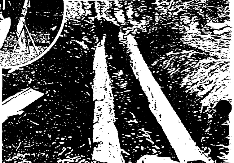
Making Culvert from Tree
