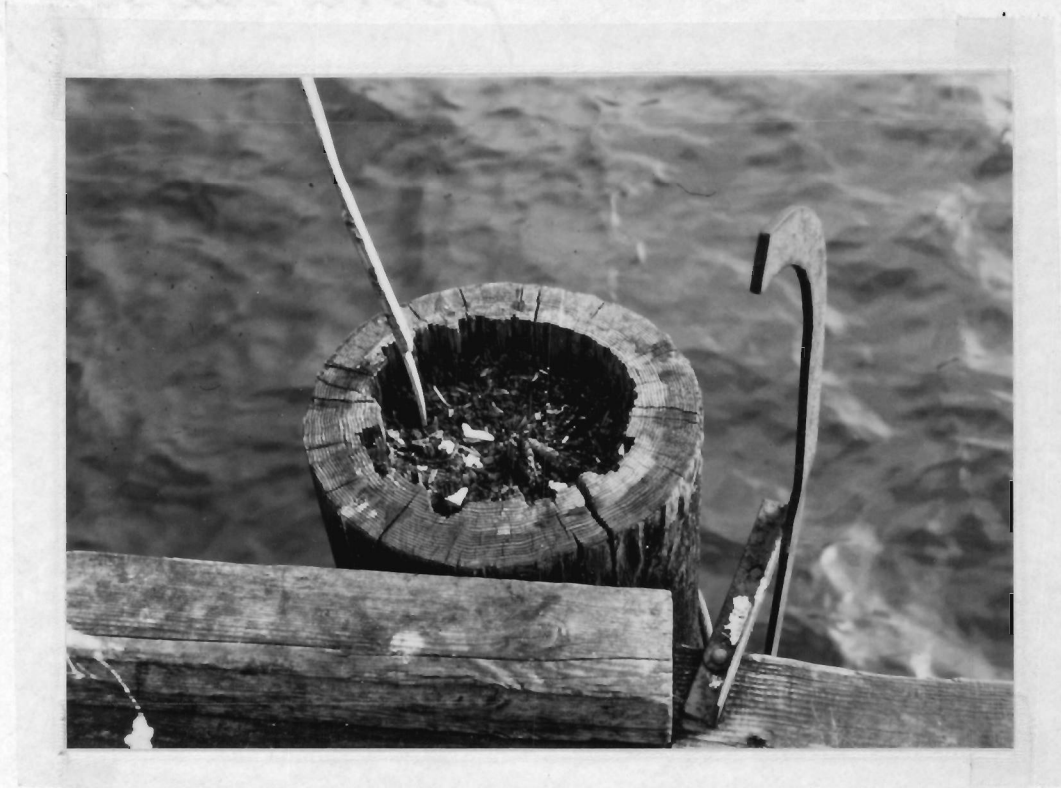
Figure 1. Top decay of piles is frequently found.
