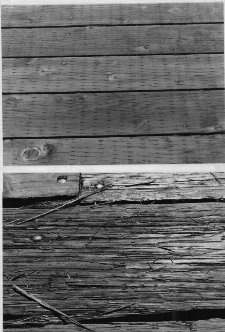
Figure 11. Decking planks treated with creosote (above) showing no surface splintering after 10 years as opposed to the surface splintering in 20-year old decking planks treated with FCAP (below).
