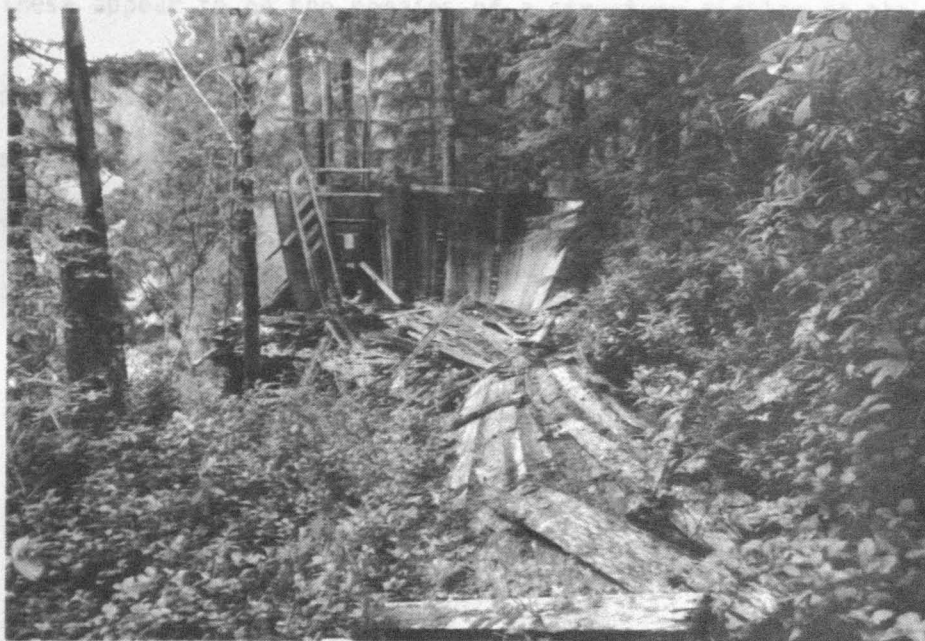
Remains of water tank with collapsed flume in right foreground.
