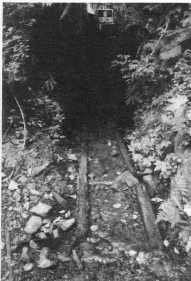
Crown Mine portal showing wooden rails
