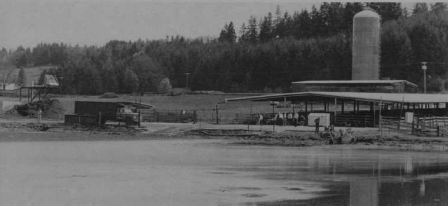
Figure 4. The lagoon in the foreground collects, treats, and stores the liquid wastes. The separation screen (left) removes the solids, which can be used as bedding material.
